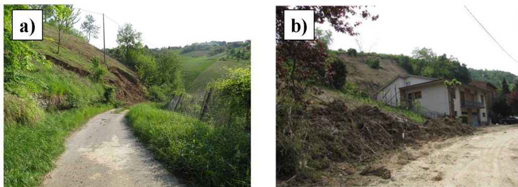
Figure 19. Shallow landslides that reached high value of IC that effectively hit the main road network during the event of 2009 in the Rio Frate catchment.
