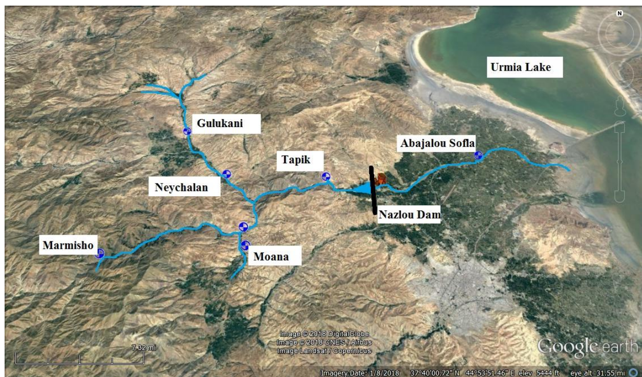
Figure 3.21. The hydrographic network and location of the hydrometric stations and of the under evaluation Nazlou Dam in the NazlouChai River catchment.
