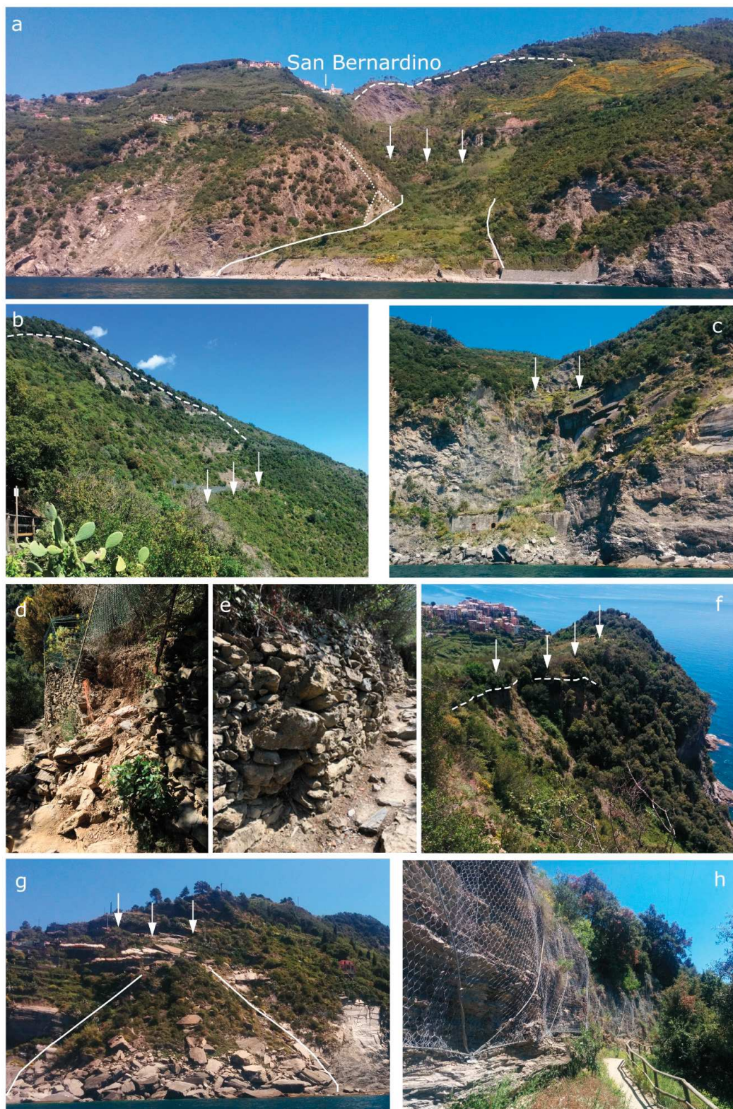
Figure 4. Main landslides and critical issues recognized along the “Sentiero Verde-Azzurro” trail: (a) Guvano landslide; (b) Macereto area; (c) rock sea cliff equipped with falling rock protections, Crovarla Valley; (d) local dry-stone wall collapse along the path; (e) visible dry-stone wall deformation along the SVA trail between Vernazza and Corniglia; (f) degradation scarp in correspondence of the Guvano beach, close to Corniglia; (g) rockslide close to Vernazza; and (h) local rock falls corresponding to the bedrock outcropping along the “Sentiero Verde-Azzurro” trail. White arrows indicate the path location.
