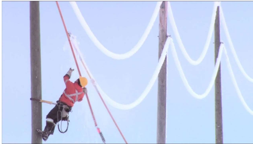
Figure 1.11 – a method of active de-icing
