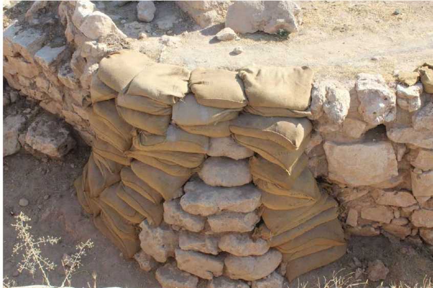
Figure 56: Both sides surrounding the retaining wall in Area J5 of the temple, with burlap bags filled with the same fallen stone accumulations. Personal photograph by the author, 2019.
