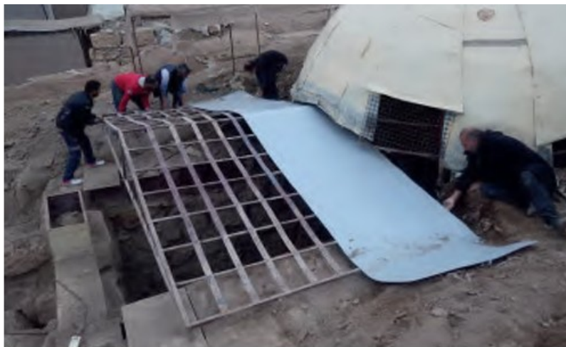
Figure 51: The new metal sheets with a fixed metal grid covering the entrance of the Abi. Source: Buccellati et al. 2018, 37.
