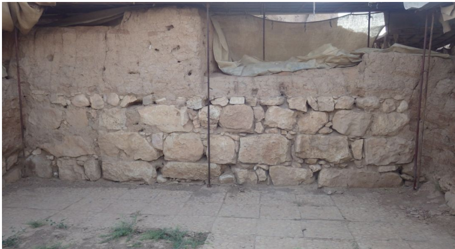
Figure 41: The eastern wall of Room D1 (D1-1) in service wing.
