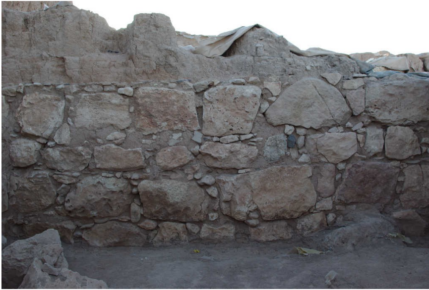
Figure 40: The large eastern wall of Room C1 (C1-1) in service wing.
