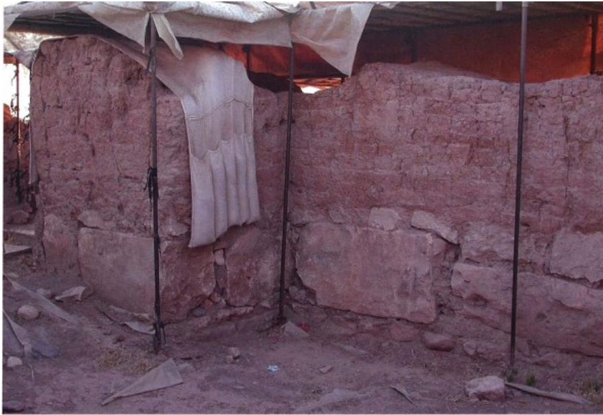
Figure 58: The reinforcement of weak walls with sand-filled saddlebags in the palace area. Source: Buccellati. 2006, 76.
