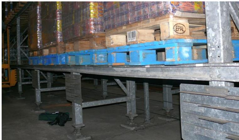
**Figure 4-3. Example of lipped channels used as pallet beams.**
