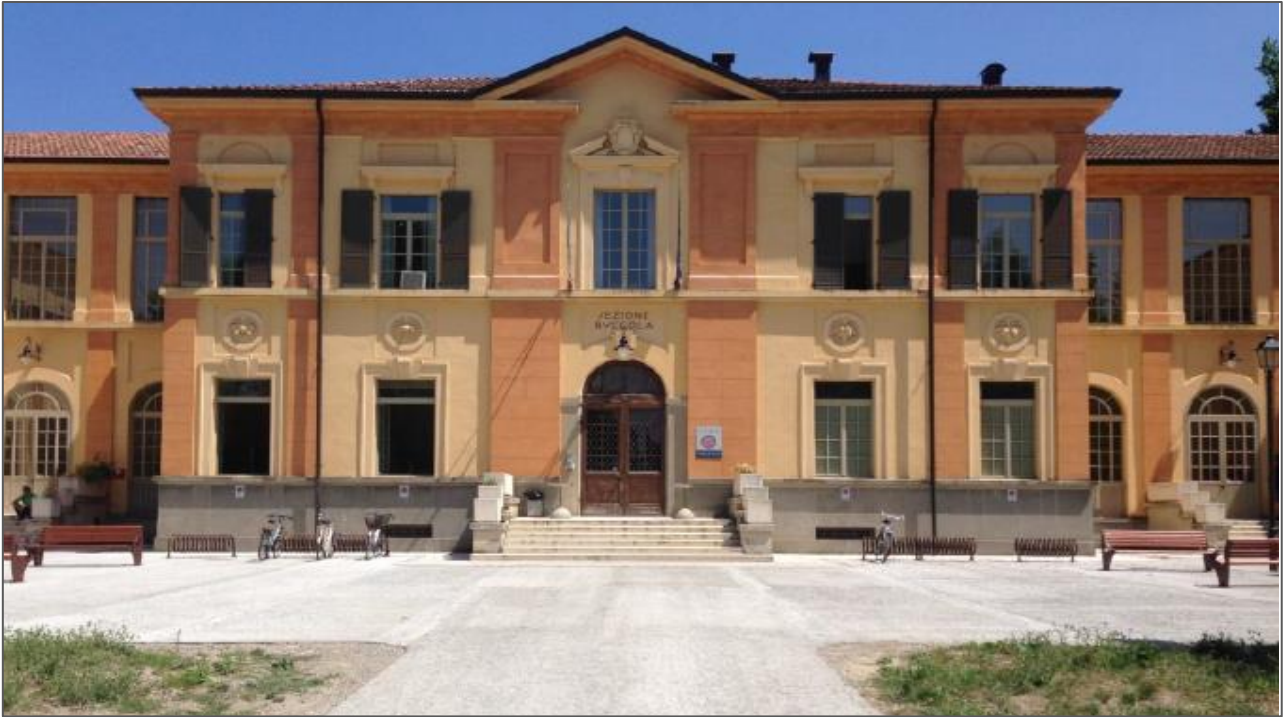
Figure 21. Buccola pavilion after the restoration intervention. Front entrance view.
