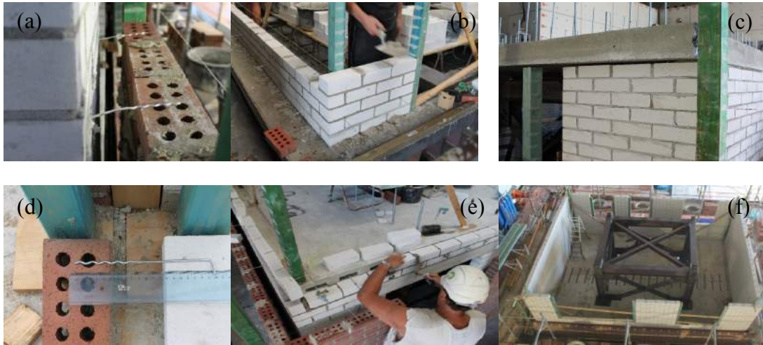
Figure 2.5 Construction details of the specimen: (a) positioning of cavity steel ties; (b) building phase of inner CS leaf; (c) laying of the second-floor slab; (d) geometry of steel tie; (e) construction of CS leaves at second floor level; (f) safety steel frame.
