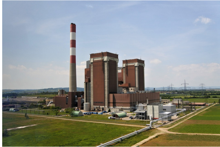
Figure 3.1.3: A picture of a thermal power plant. [Credits: free public domain images Pixabay . com]
