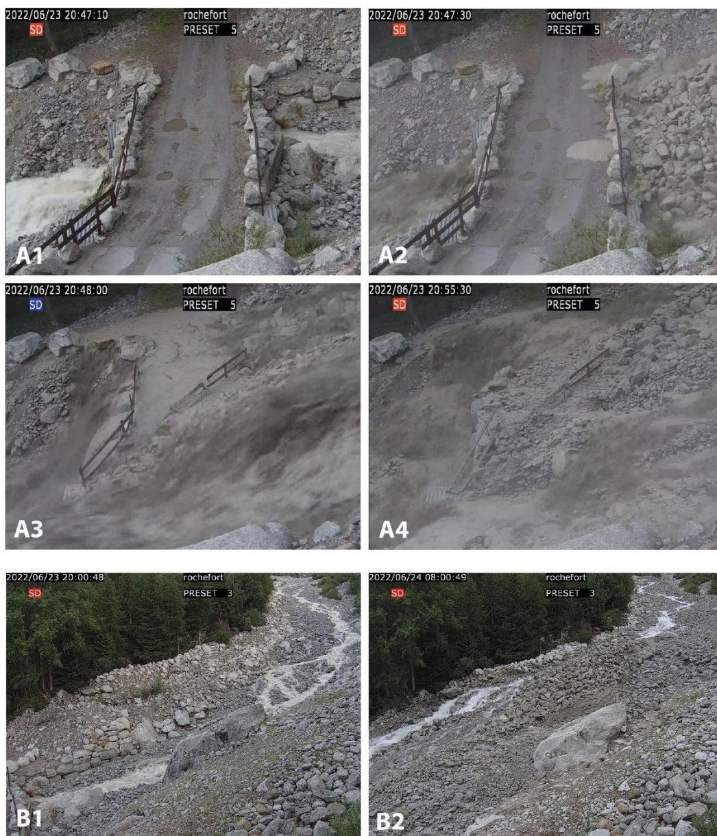
FIG. 6 - Sequence of images of the Rochefort bridge that crosses the Montitaz Stream. A1 to A4 are images of the camera surveying the bridge when the debris flow impacted the bridge h 20:47-h 20:55. B1 and B2 are images of the camera surveying the Montitaz Stream just above the bridge at h 20:00 before and at h 08:00 the morning after the event. A significant deposition of debris is evident.
